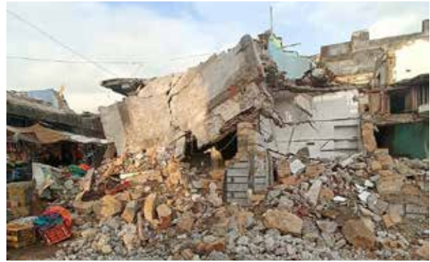
Figure 23: Demolition waste at Sant Kabir Road
