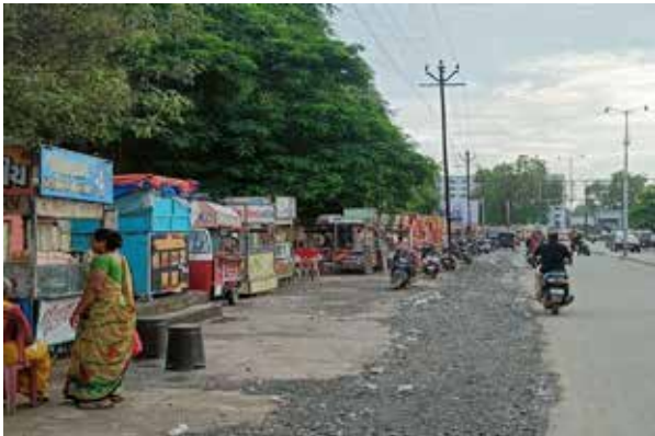
Figure 18: Lack of NMT infrastructure near College Road in Gandhi Gram
