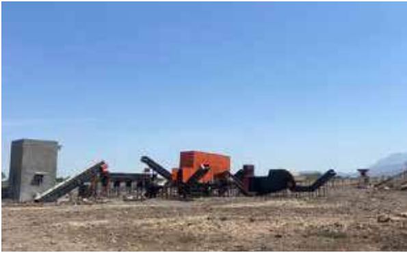
Figure 25: Auto-segregation facility at Ivnagar
